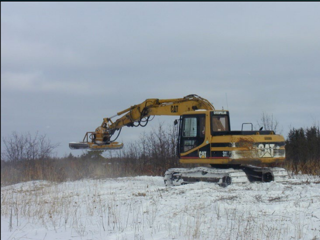
Flail Mower Excavator
