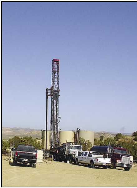
Small well pads minimize habitat disturbance at drilling sites.
