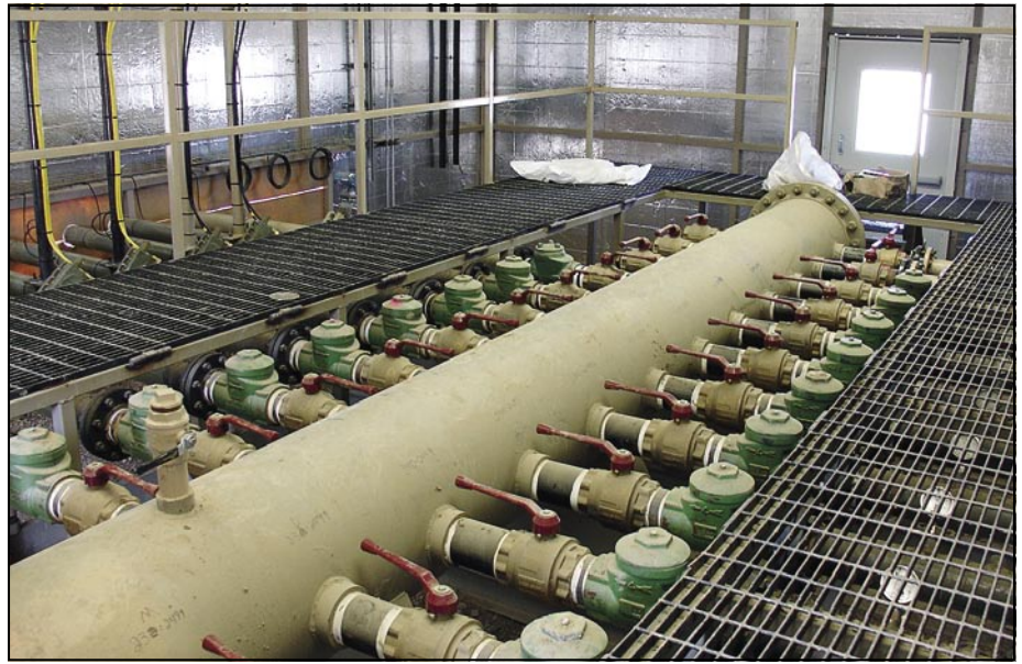
Production structures have sound-proofing insulation to reduce noise that may disturb some wildlife species.
